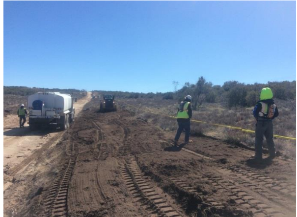
Photo 4: Archaeological and Native American monitors were present during road widening activities along McCain Valley Road in accordance with MM CUL-1D. Water was applied regularly to reduce dust in accordance with the Dust Control Plan and MM AQ-1 and disturbance limits were demarcated with yellow tape in accordance with the February 1, 2017 NTP.
