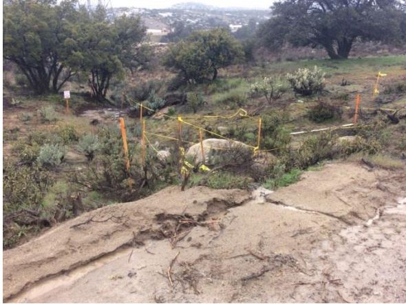
Photo 1: ECMs and SWPPP monitors observed and reported locations along McCain Valley Road where recent grading activities changed the path of overland flow and additional BMPs are required to ensure sediment remains on the ROW. Tule Wind, LLC had BMP installation and maintenance crews onsite to resolve these issues during this reporting period.
