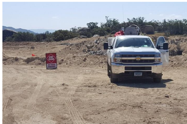
Photo 8: Fire safety coordinator and required signs were present during Hot Work at turbine pad G12 in accordance with the issued Hot Work Permit and MM-FF-1.
