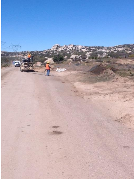
Photo 3: ECMs observed construction crews hydromulching topsoil salvage windrows along McCain Valley Road in accordance with the SWPPP.
