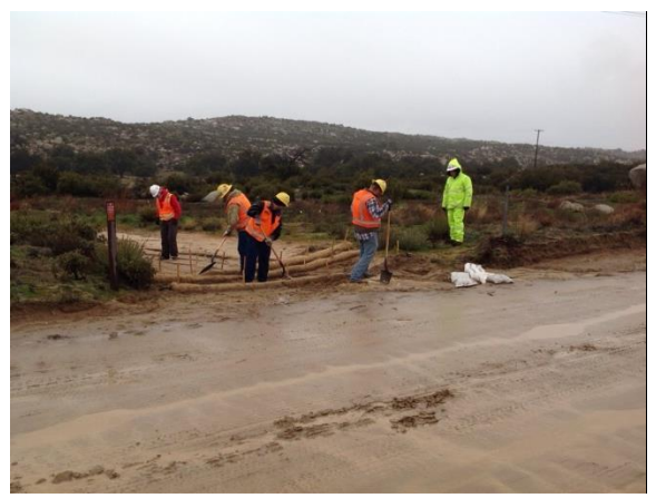
Photo 4: Crews installing additional straw wattles and maintaining existing erosion and sediment control devices along McCain Valley Road in accordance with the SWPPP and MM HYD-1. Cultural monitors were present to observe ground disturbance associated with the installation and maintenance of sediment control devices in accordance with MM CUL-1D.
