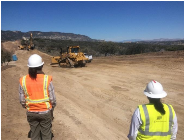
Photo 7: Archaeological and Native American monitors were present during grading activities along McCain Valley Road in accordance with MM-CUL-1D.
