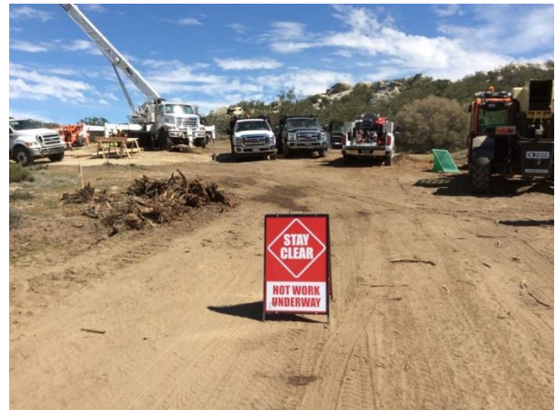
Photo 4: Required equipment and warning signs were present at the Transmission Line Pole 4 during hot work activities in accordance with the issued hot work permit and the Fire Prevention/Protection Plan (MM FF-1).
