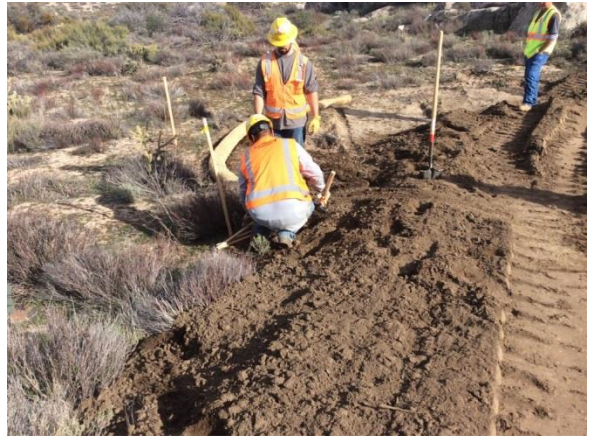
Photo 2: Crews installing additional straw wattles along McCain Valley Road in accordance with the SWPPP and MM HYD-1.
