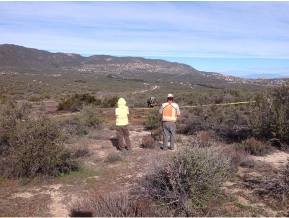
Photo 5: Biological monitors were present to observe grubbing activities in accordance with MM BIO-1C. All observed activities occurred within the disturbance limits in accordance with MM BIO-1A. Yellow tape was strung between disturbance limit stakes to increase visibility of limits for masticator operators in accordance with the NTP issued on February 1, 2017.
