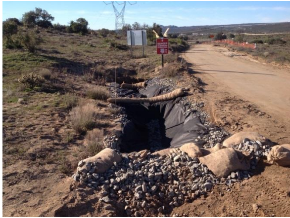
Photo 1: Crews began installing catch basins and rip-rap sediment and erosion control devices to replace damaged and failing straw wattles and sand/gravel bags in accordance with MM HYD-1 and the SWPPP. Photo shows a completed catch basin along McCain Valley Road where sediment was previously documented leaving the project site during SWPPP inspections.
