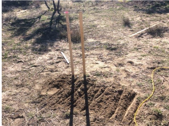
Photo 3: Spill from overturned portable sanitation facility cleaned and stained soil removed in accordance with Section 8.3 of the Hazardous Materials Management Plan. Tule Wind LLC is working to determine a permanent solution to securing the portable sanitation facilities onsite.
