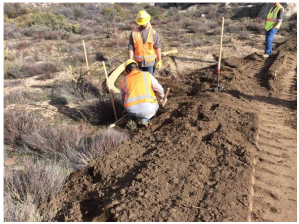
Photo 4: Crews installing additional straw wattles along McCain Valley Road in accordance with the SWPPP and MM HYD-1.
