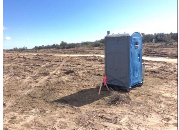
Photo 2: The portable restroom which had blown over during a period of high winds on February 27, 2017 was turned upright and staked the following day to prevent the issue from reoccurring. The stained soil was removed in accordance with MM HAZ-1A.
