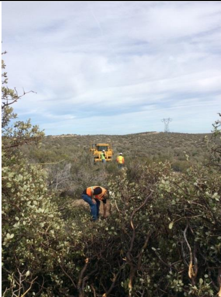
Photo 3: Resource monitors and equipment operators cut pre-grubbing lines in thick vegetation along the yellow tape disturbance limits with monitors acting as spotters ahead of the equipment in accordance with the February 1, 2017 NTP.
