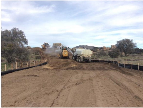
Photo 1: Clearing and grading activities observed within the staked limits of disturbance in accordance with MM BIO-1A. Water trucks in use for dust control in accordance with MM-AQ-1.
