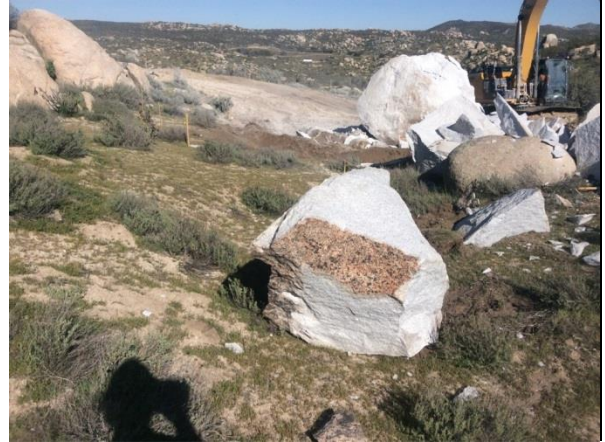
Photo 2: During blasting activities on March 16, 2017, rock debris fell approximately 10 feet outside the staked disturbance limits. The pieces of rock were left in place to avoid creating additional unauthorized disturbance.
