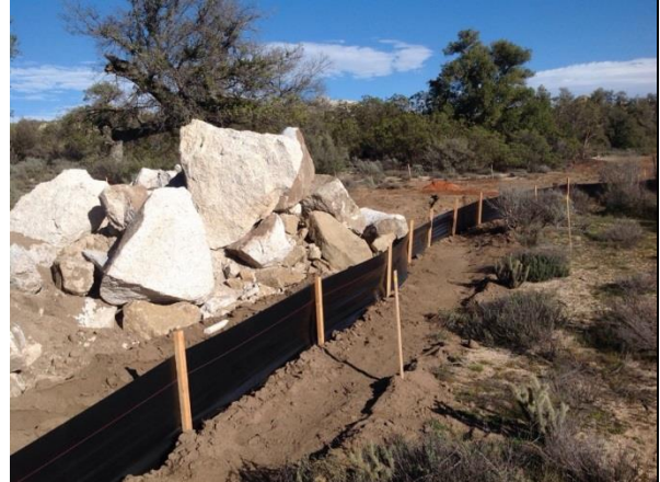
Photo 2: During this reporting period, crews repaired a damaged silt fence on the McCain Valley cutoff road per direction provided by the QSP and ECMs in accordance with the SWPPP.
