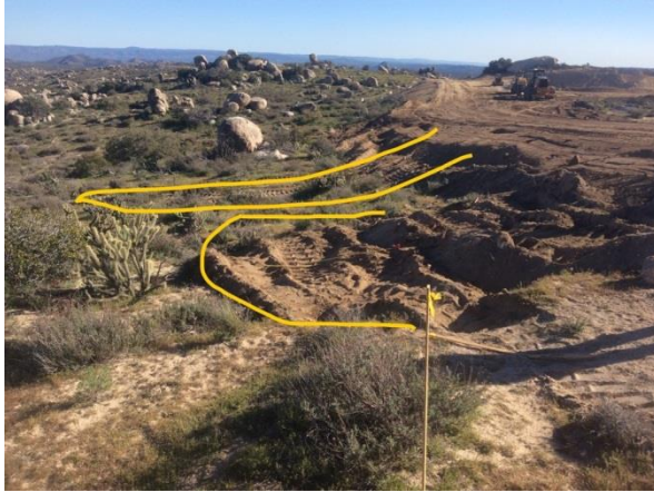
Photo 1: On March 13, 2017, disturbance beyond the staked limits of disturbance occurred when a piece of construction equipment hit a subsurface rock and lost control. The area of disturbance was inspected and it was determined that no damage to sensitive environmental resources occurred.
