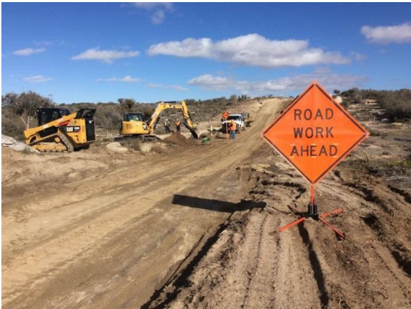
Photo 1: ECMs and SWPPP monitors observed and reported locations along McCain Valley Road where recent grading activities changed the path of overland flow and additional BMPs are required to ensure sediment remains on the ROW. Tule Wind, LLC had BMP installation and maintenance crews onsite to resolve these issues during this reporting period.
