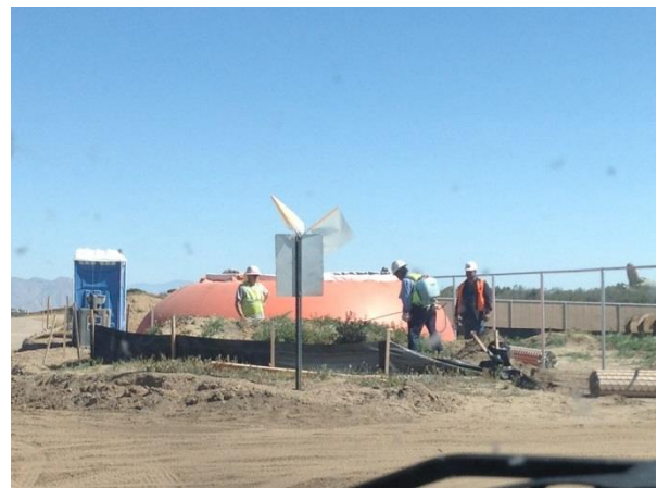
Photo 4: During this reporting period, herbicide was applied along the E String by a QAL holder and under the supervision of a Habitat Restoration Specialist, in accordance with Section 6.1.2 of the Habitat Restoration Plan.
