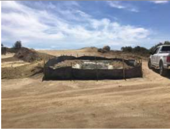
Photo 1: ECMs confirmed that the silt fence surrounding the concrete washout at turbine pad G15 was repaired and a rock apron was installed in accordance with the grading plan design detail WM-8.
