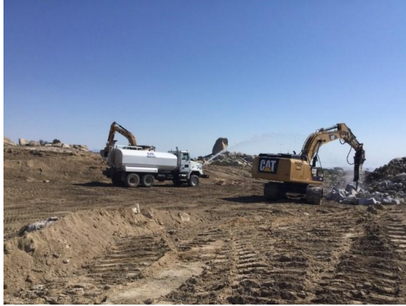
Photo 1: Rock-breaking activities observed within the staked limits of disturbance in accordance with MM BIO-1A. Water trucks are present for dust control in accordance with MM-AQ-1 and MM-FF-1.
