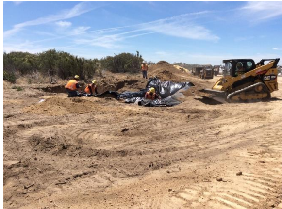
Photo 4: The new concrete washout pits at Yard 6 were double-lined with thick poly sheeting to prevent soil contamination in accordance with MM HYD-1 and the project SWPPP.
