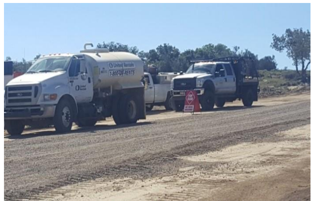
Photo 8: Fire safety coordinator, a water truck, and required signs were present during hot work activities in accordance with the issued Hot Work Permit and MM-FF-1.
