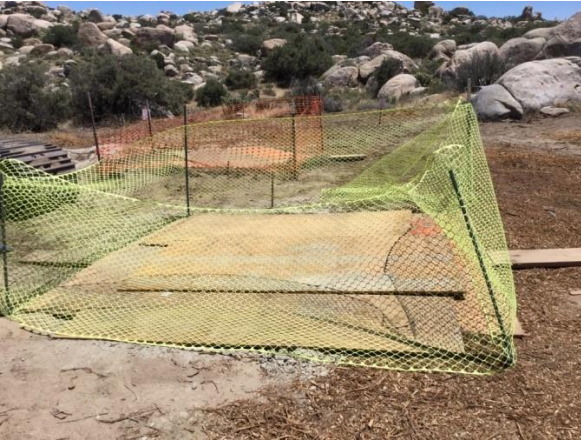
Photo 5: Excavations are covered to prevent wildlife from becoming entrapped in accordance with MM-BIO-7A.
