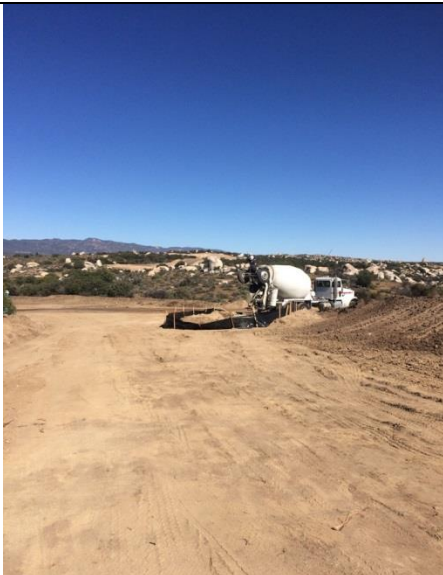
Photo 3: ECMs observed the concrete washout at turbine pad G15 without a rock apron as required by design detail WM-8 included in the grading plans. ECMs notified Tule Wind, LLC of the problem area. A rock apron is anticipated to be installed in accordance with the grading plans.
