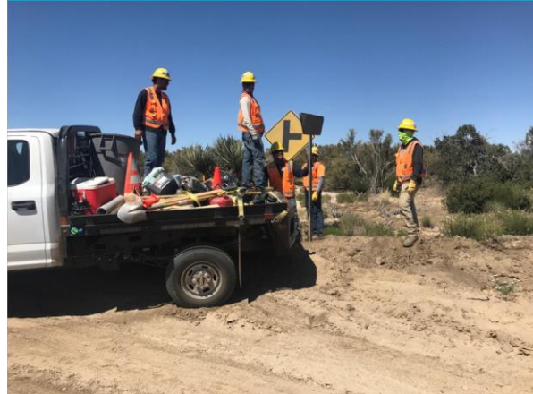
Photo 6: Construction crews replace and re-install traffic signs along McCain Valley Road in accordance with the Traffic Control Plan (MM-TRA-1).
