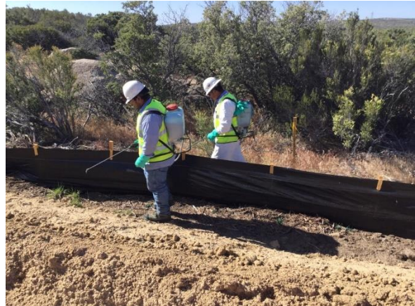
Photo 2: Crew spraying herbicide within disturbance limits on A string. A qualified restoration monitor was present per MM BIO-3A.
