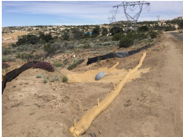
Photo 3: Erosion blankets and biodegradable straw wattles are installed along culverts in accordance with MM-HYD-4 and site specific SWPPP.
