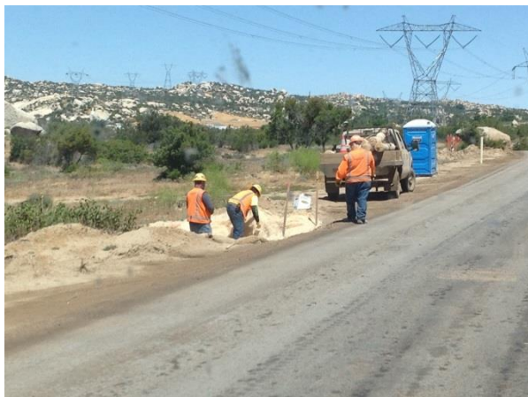
Photo 3: Erosion control devices were installed at culverts along McCain Valley Road in accordance with the project SWPPP.
