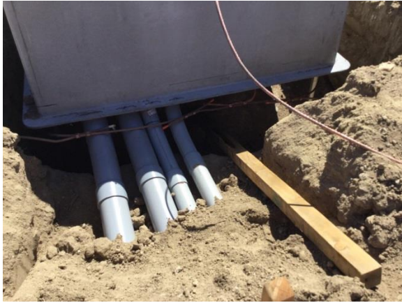
Photo 1: ECMs confirmed that wildlife ramps were installed in the open excavation at turbine site G11 in accordance with MM BIO-7A.
