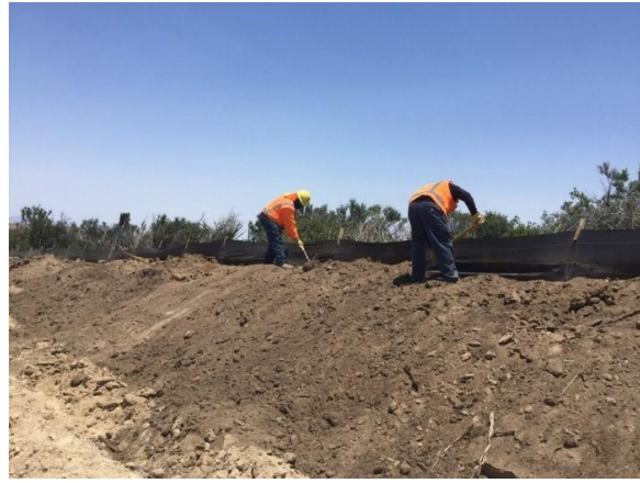
Photo 2: Construction crews are observed replacing silt fencing along the D1 access road in accordance with MM-HYD-1 and the project specific SWPPP.
