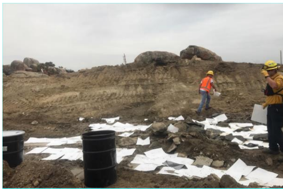
Photo 3: On 5/31/2017, construction crews are observed using absorbent materials to address a hydraulic leak per MM-HAZ-1a and the Hazardous Materials Management Plan.
