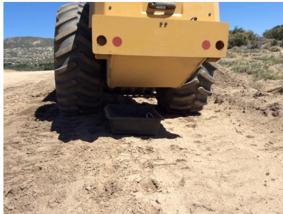
Photo 4: ECMs observed containment bins beneath parked equipment to prevent potential leaking equipment from staining soils in accordance with MM HAZ-1A and the Hazardous Materials Management Plan.
