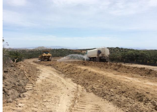
Photo 4: ECMs observed road grading on the access road between pad sites C2 and C5 with an accompanying water truck in order to minimize fugitive dust as per MM AQ-1. Yellow tape is shown marking limits of disturbance in accordance with the February 2, 2017 NTP.
