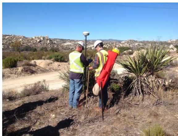
Photo 4: Westwood survey crews staking limits of disturbance along McCain Valley Road in accordance with MM BIO-1A.
