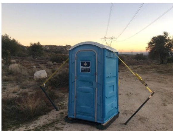
Photo 5: Portable restroom facilities are staked to the ground surface with containment in place to prevent the potential for leaks or spills in accordance with ROW Grant Stipulation 78 and the HMMP.
