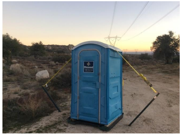
Photo 2: Portable restroom facilities are staked to the ground surface with containment in place to prevent the potential for leaks or spills in accordance with ROW Grant Stipulation 78 and the Hazardous Materials Management Plan.
