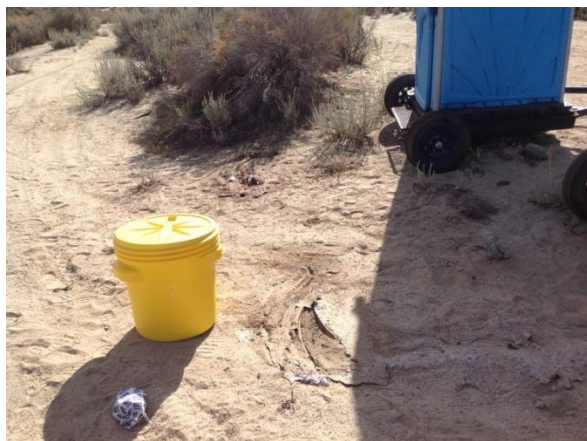
Photo 3: Spill kits were used to clean up the spill from overturned portable sanitation facilities in accordance with the SPCC and HMMP.
