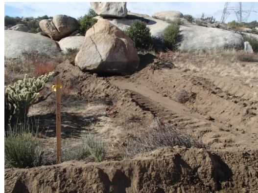
Photo 4: A boulder was pushed approximately 15 feet outside of the limits of disturbance. This event is being classified as a "Problem Area" in accordance with 5.2 of the ECCMP.
