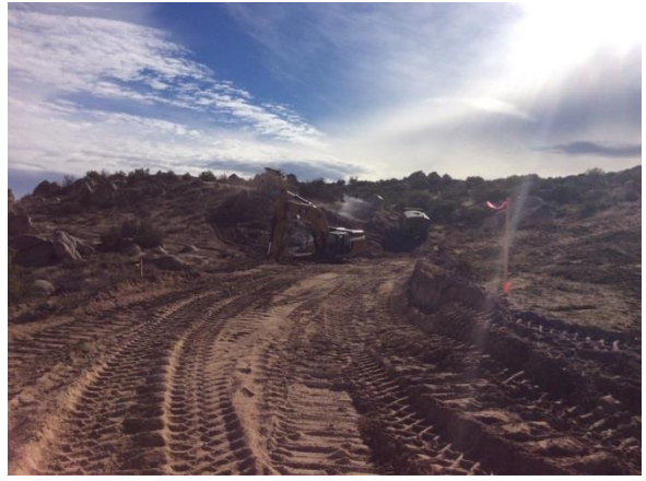
Photo 2: Clearing and grading activities observed within the staked limits of disturbance in accordance with MM BIO-1A.
