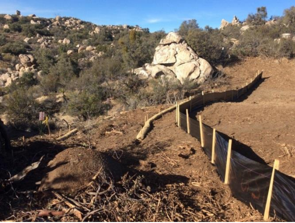
Photo 1: Erosion and sediment control devices properly installed in accordance with the SWPPP.
